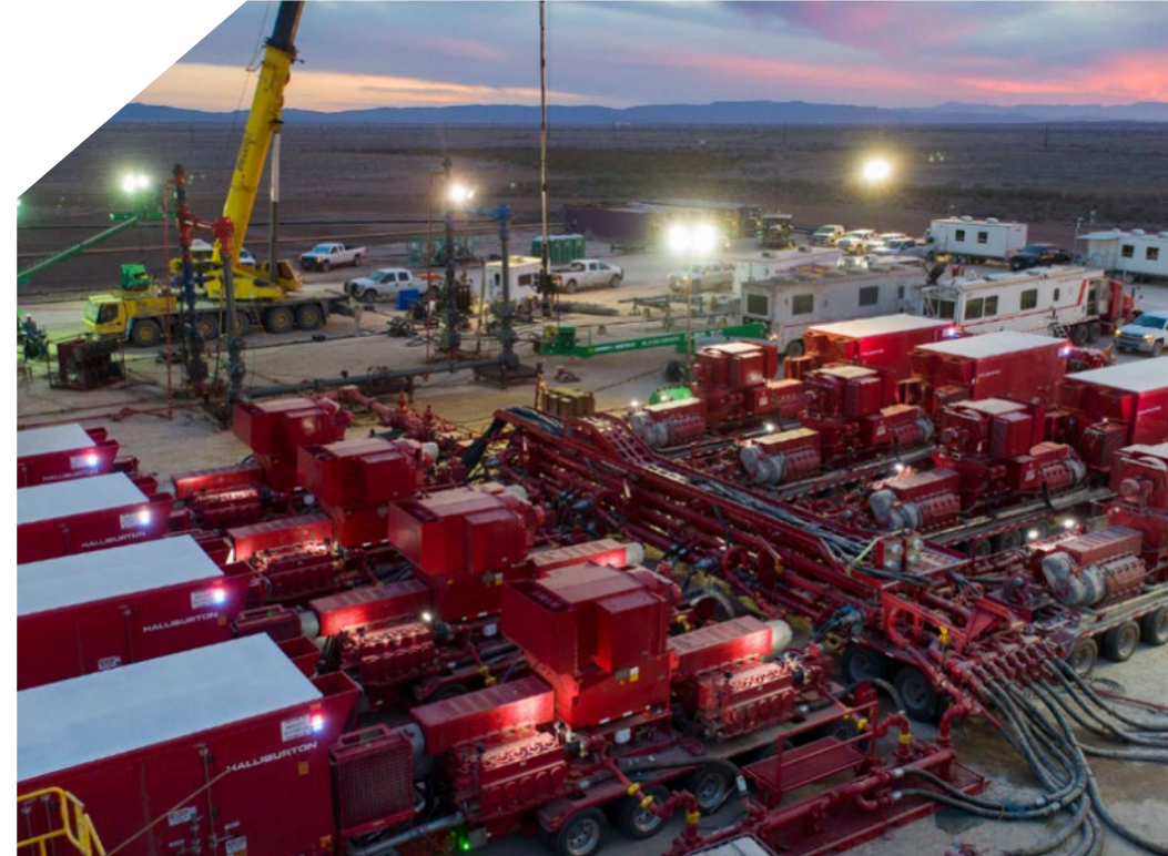
The First Fully Electric 40,000-HHP Frac Site
